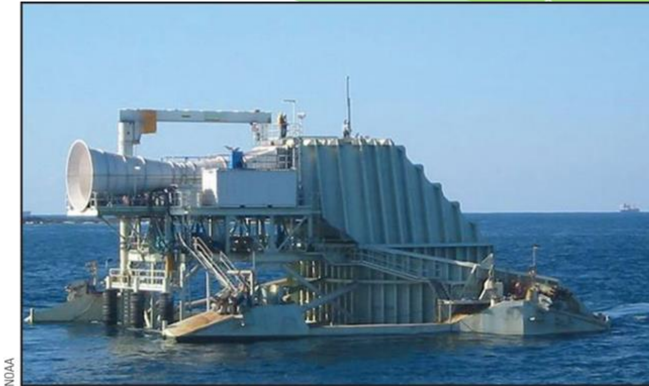
Figure 12.4: Oscillating water column developed by Energetech in Australia that is anchored near shore, rated at 500 kW.
